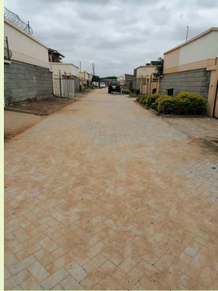
Paving access road Mombasa
