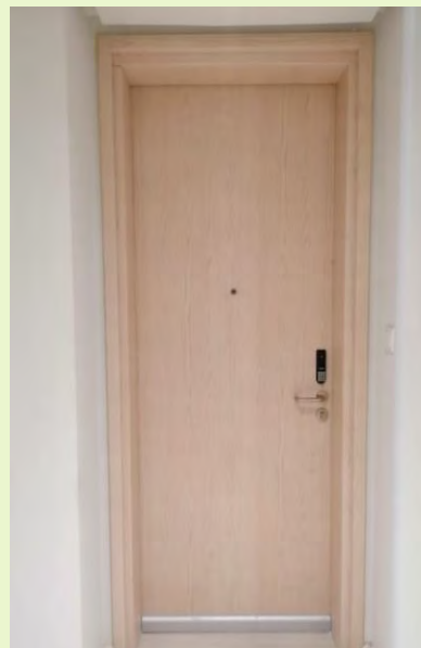
Installed Fire door and accessories Kilimani Project
