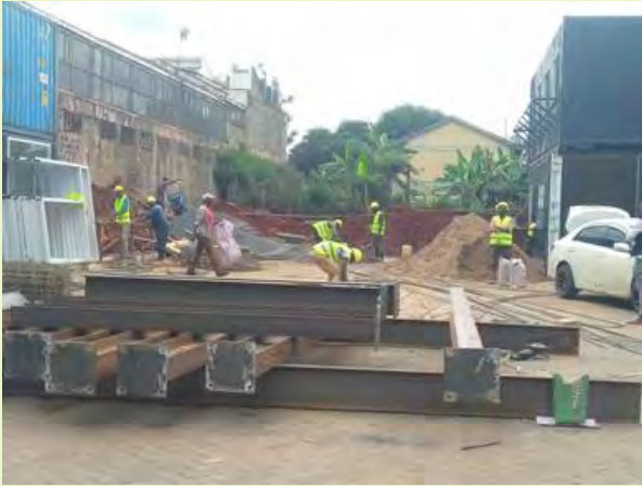
Steel fixing at Gigiri Project
