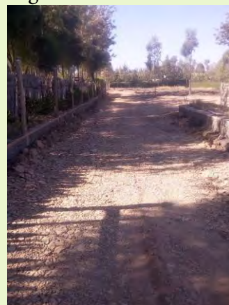
Paving access road covenant Guest House
