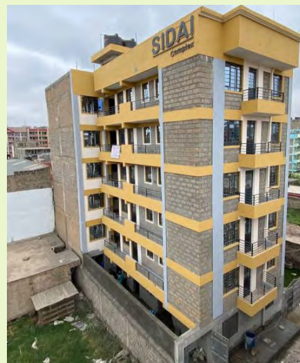
Completed Tassia Flats
