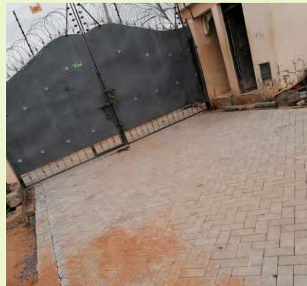
Paving access road Mombasa
