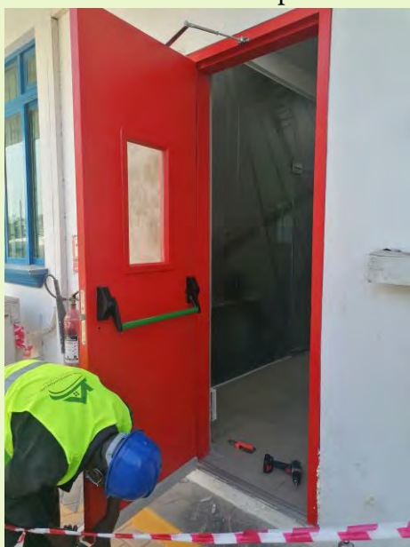
Fire Door Installation Mombasa KPA
