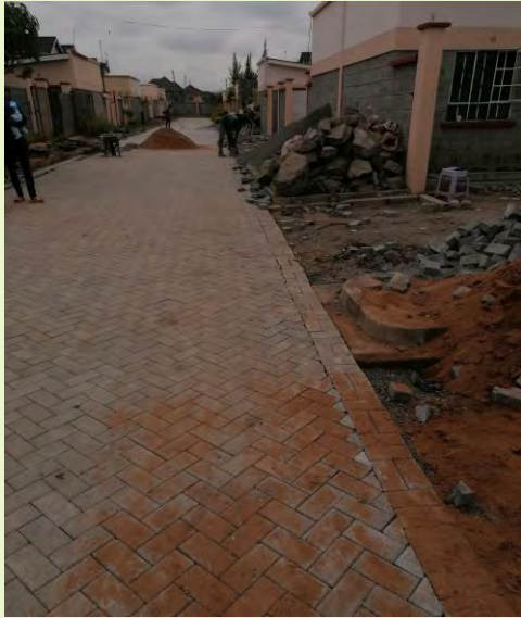
Paving access road Mombasa
