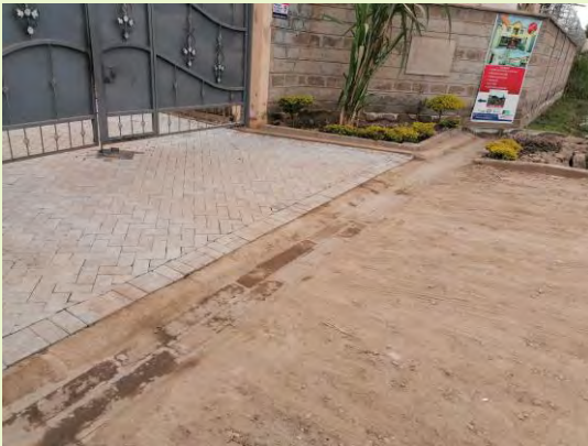
Paving access road Mombasa
